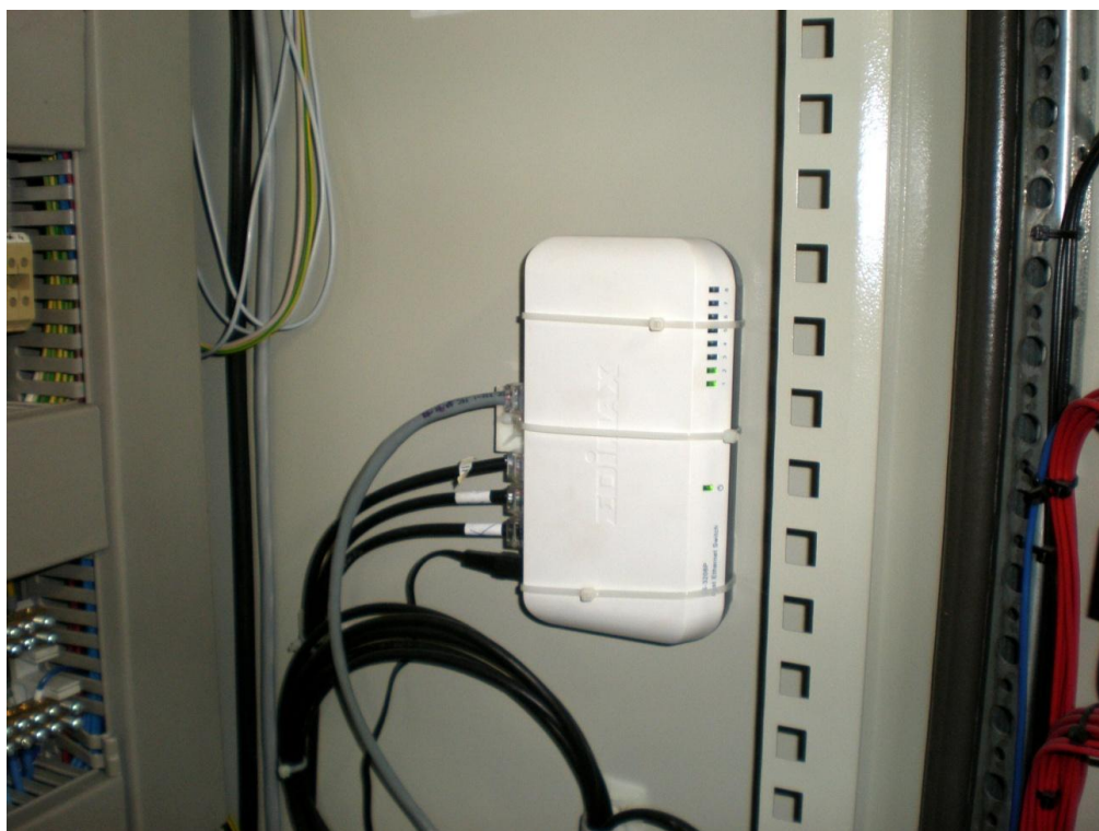
Obr. 29: Switch Edimax
